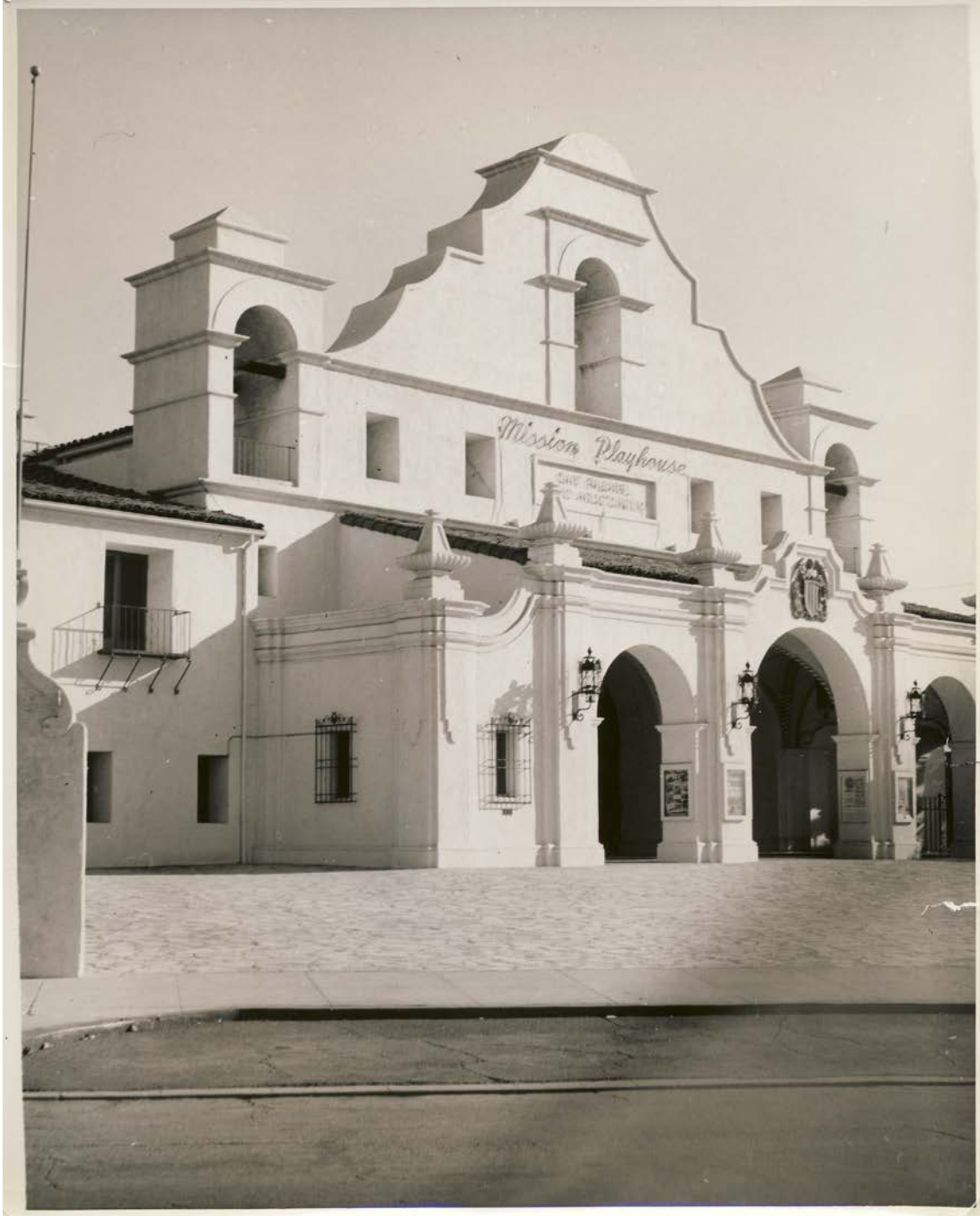
Figure 2 of 10 San Gabriel Mission Playhouse, San Gabriel, Los Angeles County, CA Photographer: unknown Date Photographed: 1927 Description: Main/south Façade, camera facing northeast
